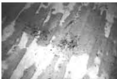
In this photo, mold growth on the slab following the removal of the floor covering, which then is allowing the surface to dry out again.
