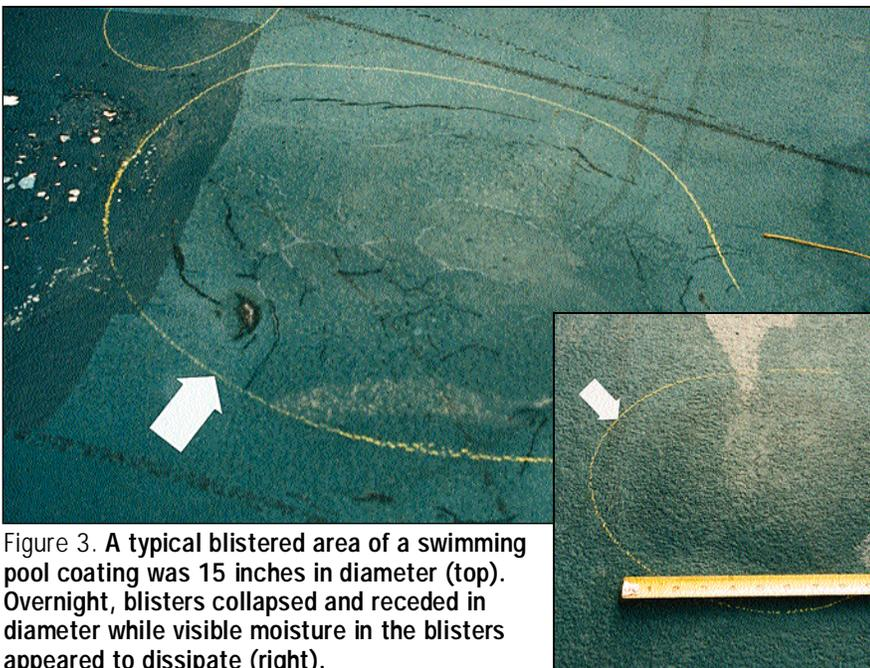
Figure 3. A typical blistered area of a swimming pool coating was 15 inches in diameter (top). Overnight, blisters collapsed and receded in diameter while visible moisture in the blisters appeared to dissipate (right).
