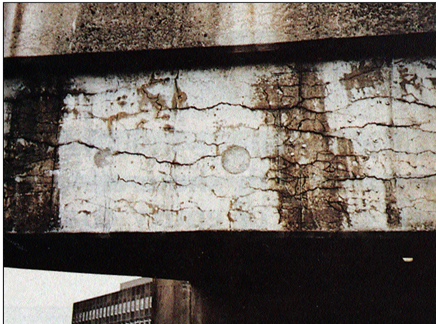
Cracking caused by alkali-silica reaction (ASR) occurs in beams, foundations, and other structures exposed to moisture. Although the width of ASR cracks may exceed 4 mm (0.16 inches), crack widths are generally less than 1 mm (0.04 inches).
